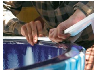
Installation of GORE® Gasket Tape Series 1000
